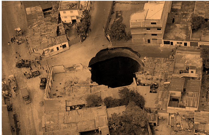
Image 2: Sinkhole in Guatemala.
